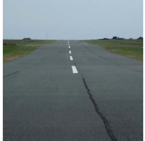
Runway 08/26 – view east from 08 Threshold accentuates undulation of existing surface
