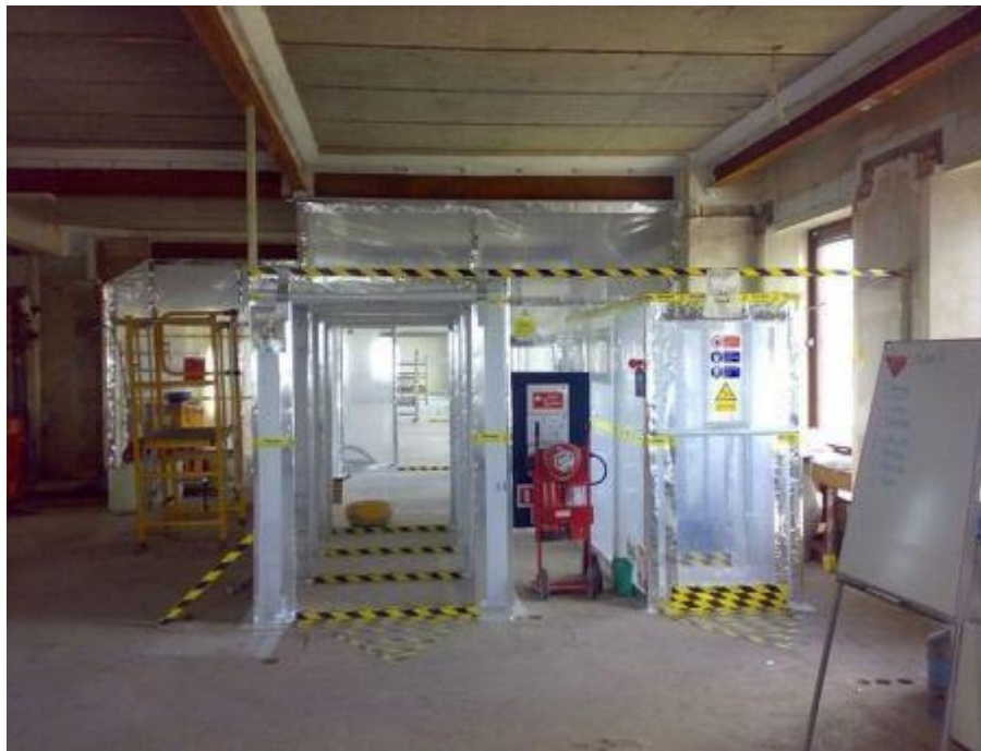
Figure 3 – Typical asbestos removal enclosure
