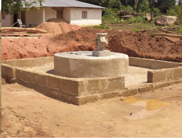
Newly constructed well awaits connection of pump before being commissioned
