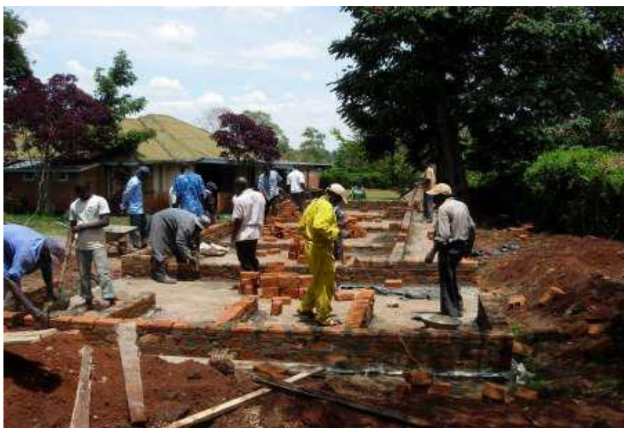
Picture 6 – Construction work on the foundations for the new hospital wards
