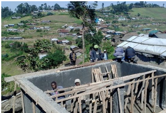
Building the storage tank
