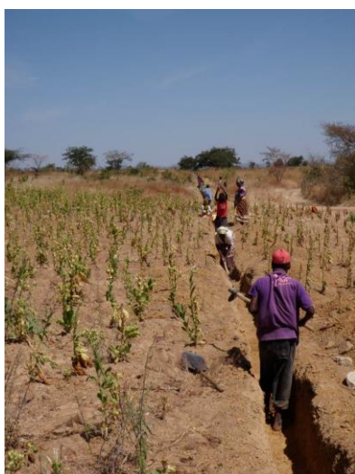
Supply pipeline trench excavation
