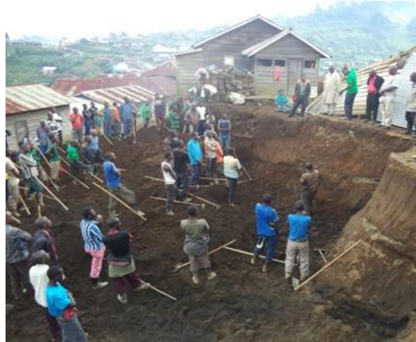
Digging the foundations for the storage tank
