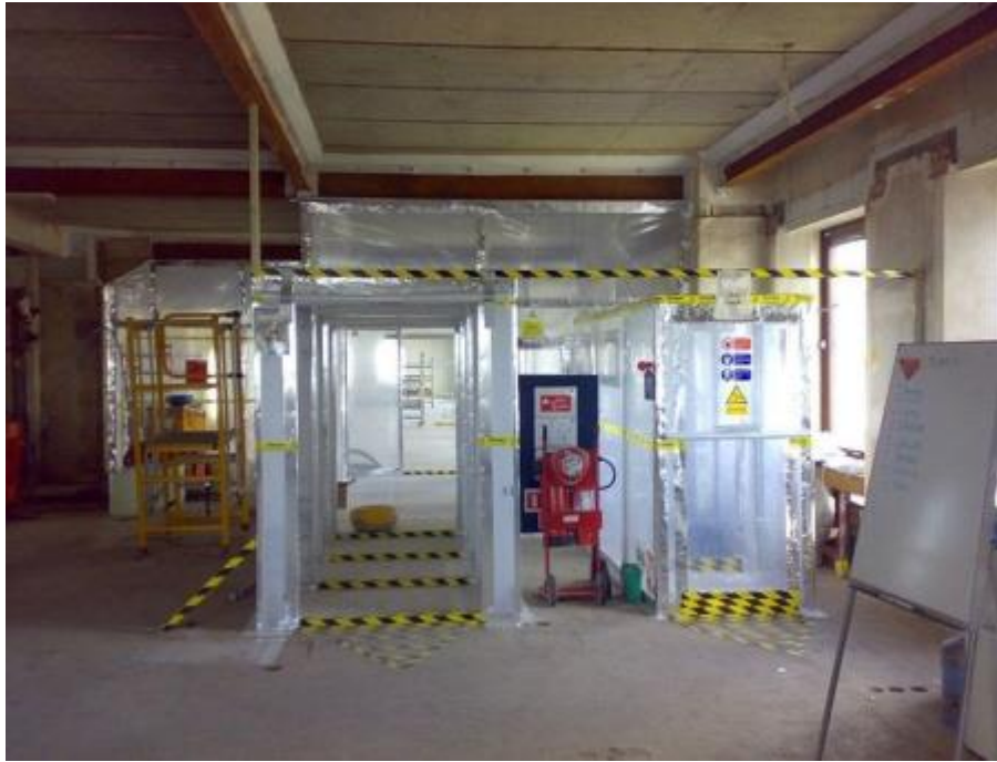
Figure 3 – Typical asbestos removal enclosure
