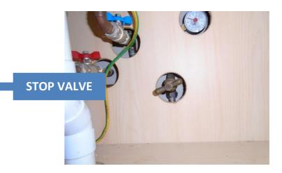
To shut off the water turn the valve clockwise until it shuts the water off. There will still be water in the water pipes, so you will need to turn on your taps to drain all the water out of the pipes. This should stop the leak until it can be fixed.
