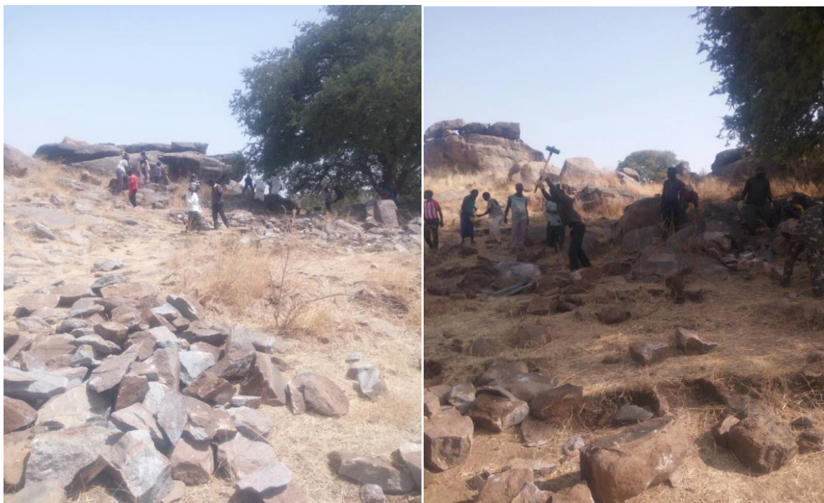
Collection and preparation of stone for the dam's walls
