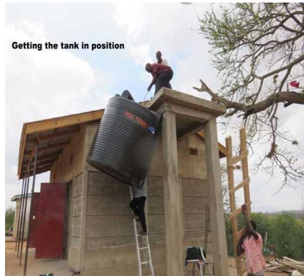
Manoeuvring the 10,000l storage tank for the new shower block into position
