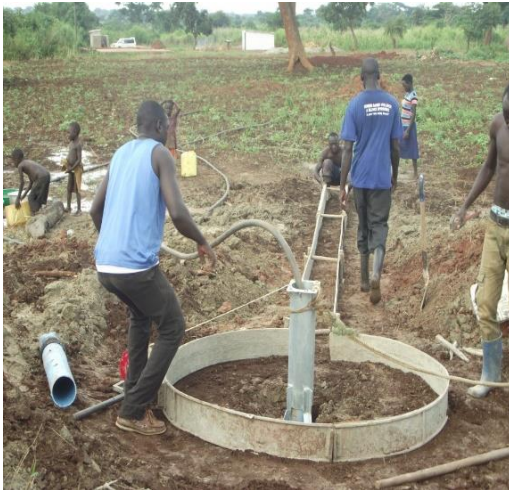
Construction of borehole
