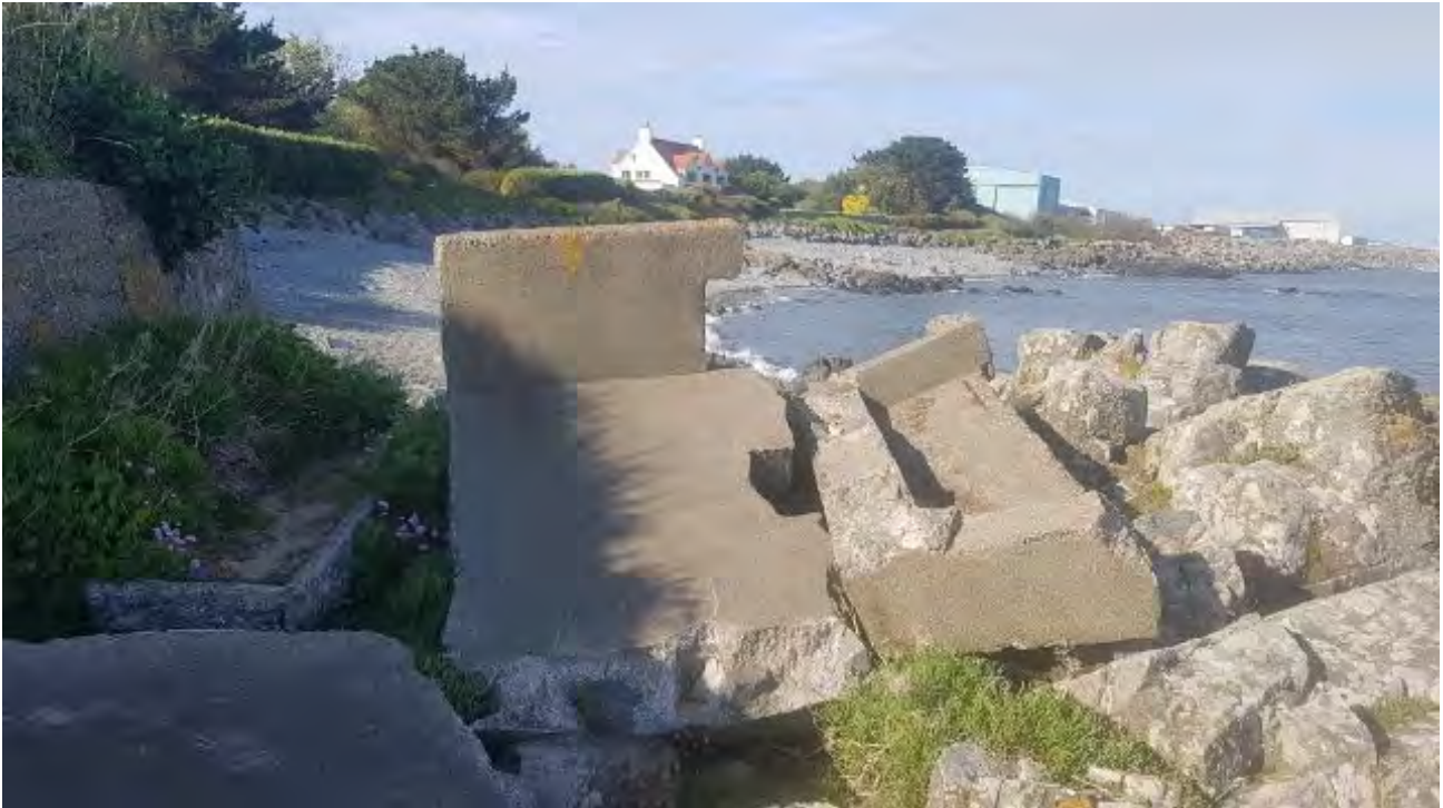
Figure 15-10 Masonry on the Foreshore Associated with MGU664, Collapsing onto the Beach
