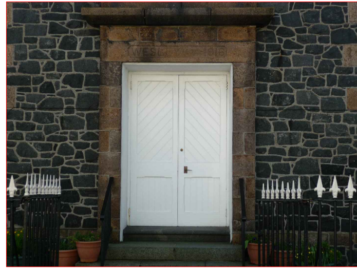
Church Entrance Doors (1)
