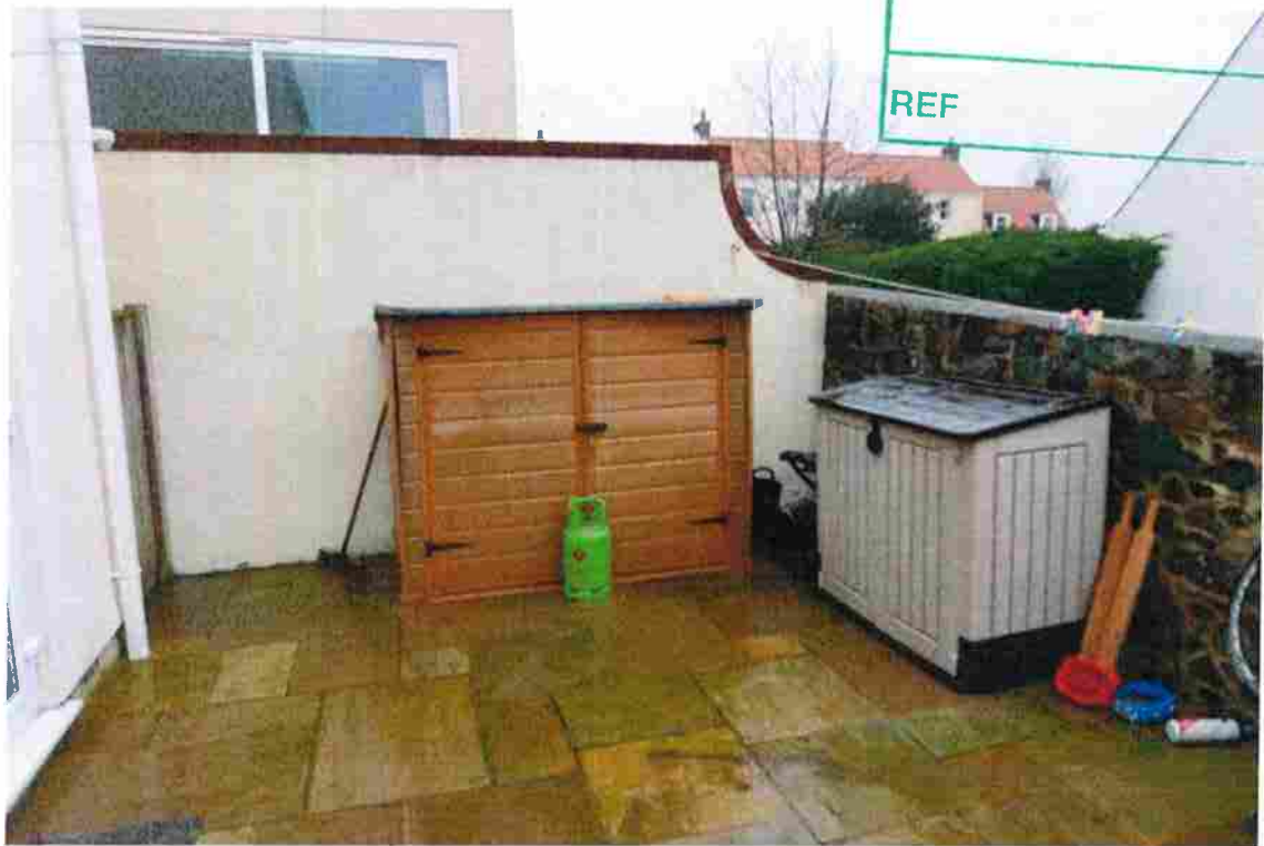
Photograph 3 – Rear Garden (Wall 1 and Wall 2 intersect)
