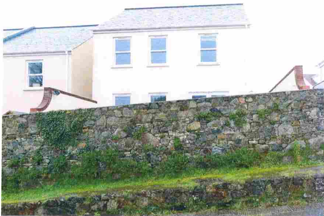
Photograph 5 – Rear Elevation (Wall 2)
