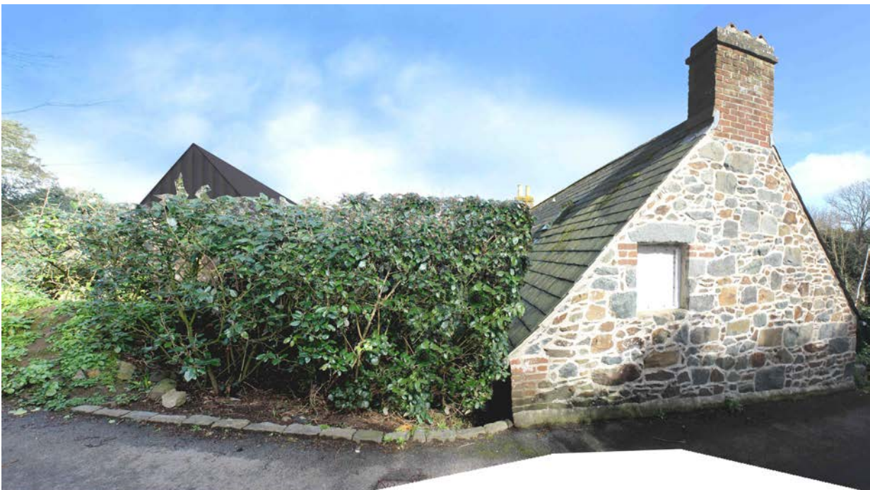
View 4 - South elevation (from road)
