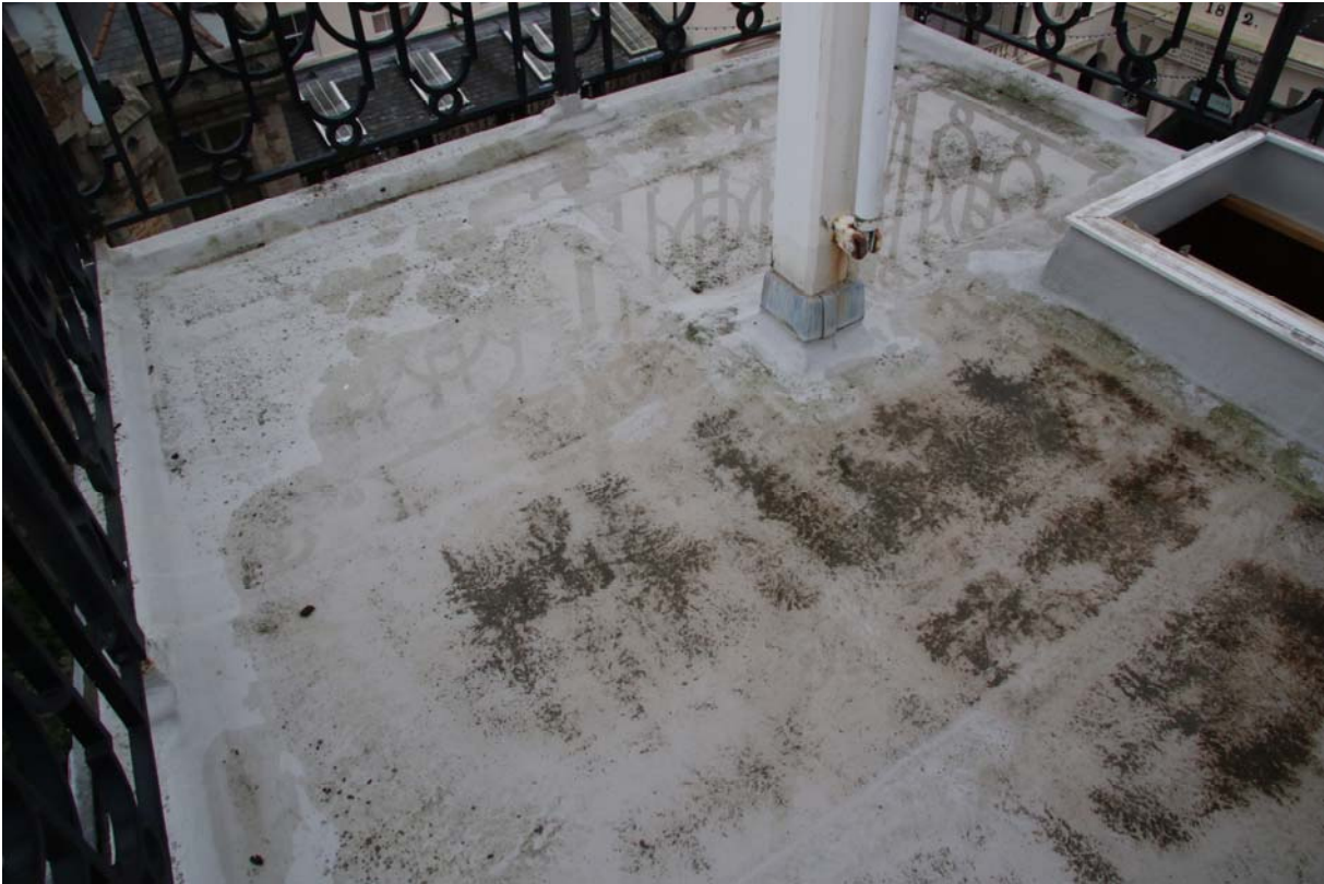
Story Tower roof – photograph 1
