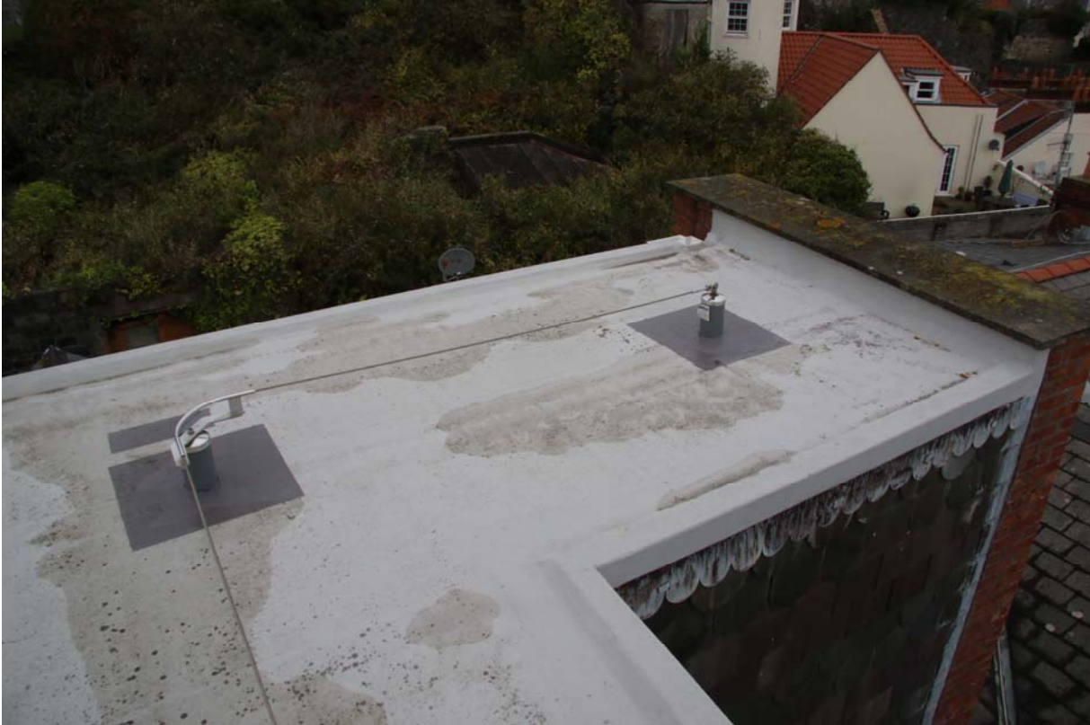
Story Tower roof – photograph 2
