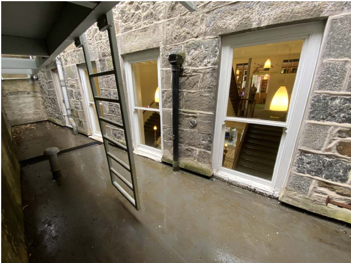
Store Room roof – photograph 1
