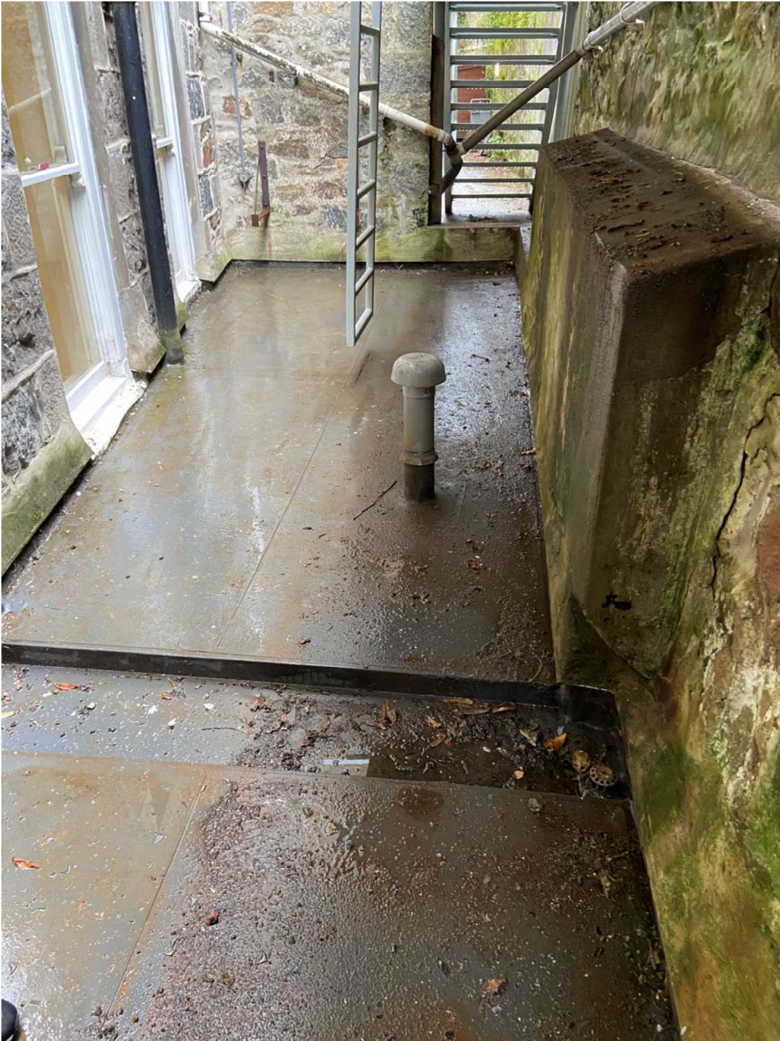
Store Room roof – photograph 2
