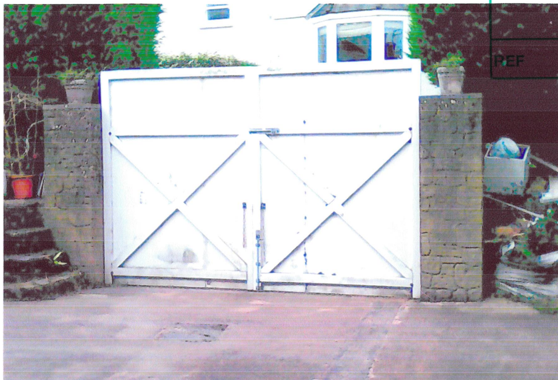
FIGURE 3B Photograph of Existing Gates and Steps to Lawn
