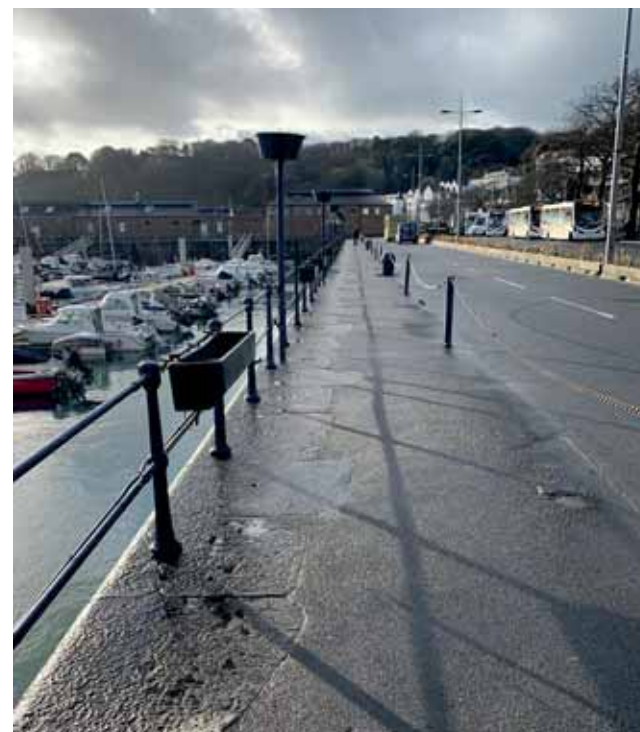
Image D.3: The harbour-side footway along South Esplanade has no kerb and only a post-and-chain barrier between pedestrians and traffic making it feel unsafe and inhospitable, particularly at night
