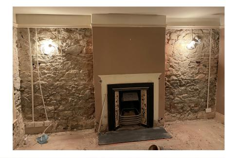
Removal of internal render (for replacement with a lime-based render – agreed Class 3 Exemption) necessitated removal of the fireplace which we had intended to reinstate along with replacement of tiles which were cracked. On commencing removal it was found that the fireplace is damaged and not able to be repaired. We therefore request permission to replace the fireplace unit with a similar unit, either reproduction or restored. Please see photos below.
