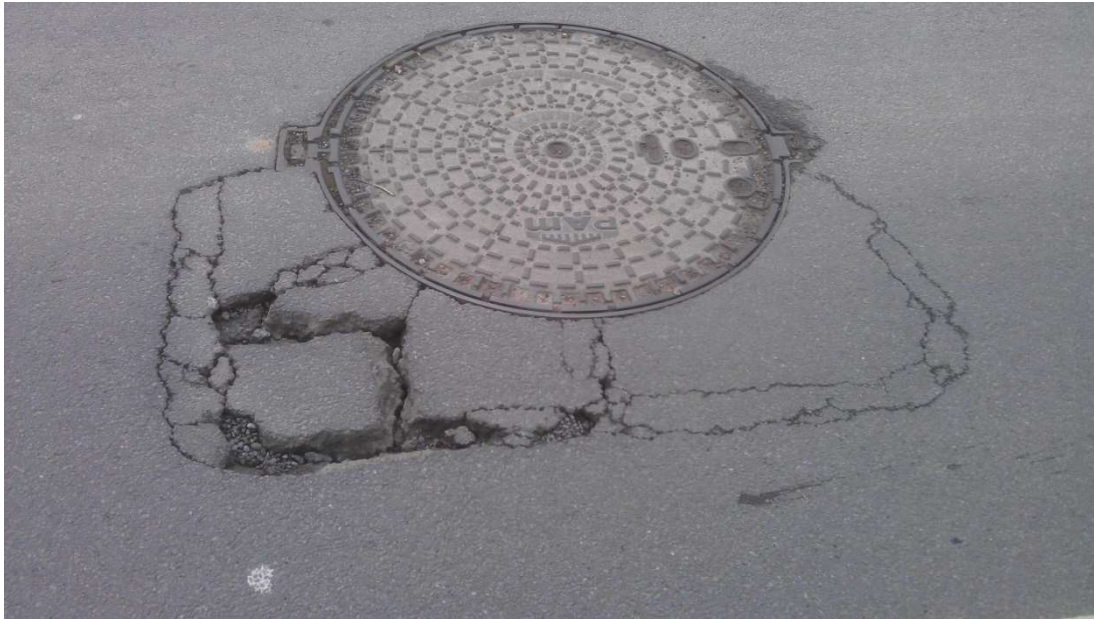
Figure 1: Cover with failed surround
