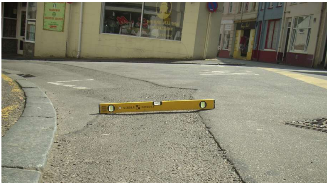
Figure 2: A subsided reinstatement
