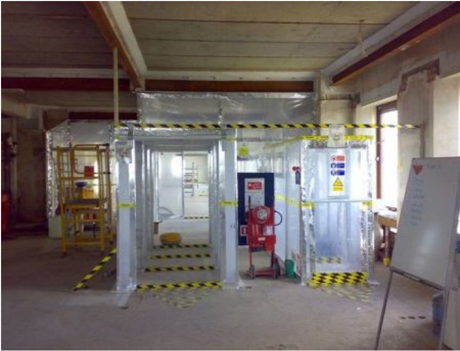
Figure 3 – Typical asbestos removal enclosure
